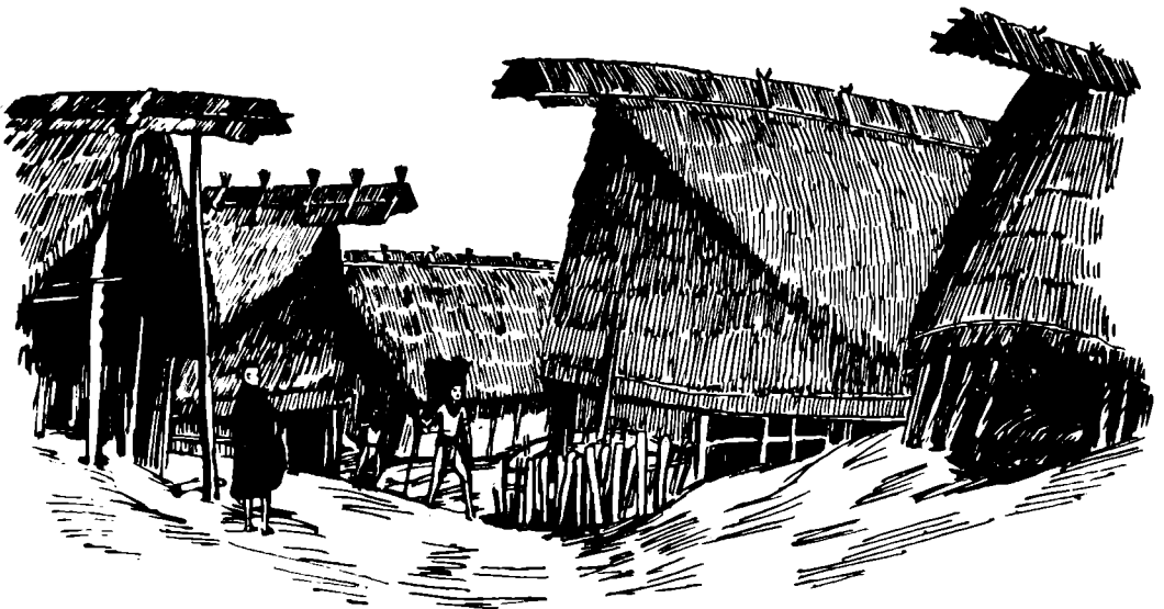
Street in Ungma village (after Mills, 1926)
